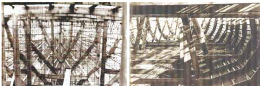
Fig. 2: Illustration of the open-mold method of construction with successive wood frames used to provide the shape of the hull
